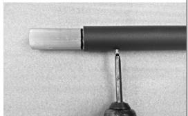
3. Measure and cut, if required, the next piece of ADA rail to be installed. Install the next piece of the rail over the remaining exposed end of the connector until the two pieces of ADA rail meet, and there is no gap between the ends of the rails. A rubber mallet may be needed to tap parts in place.
