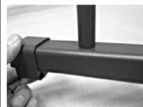
6. The 200 Series deck rail can be installed with or without a deck board on top of the top rail (A). If installing without a deck board on the top rail, measure up 35 1/4" (36" rail height) or 41 1/4" (42" rail height) from the floor and mark a level, horizontal line on the post or wall.
