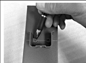
8. Attach both saddle brackets (C) with self-drilling screws (H) at the marked screw locations completed in Step 7. Pre-drilling is recommended.
