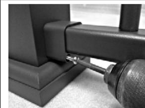
12. Screw self-drilling screws (H) into the top rail (A) from the underside of each saddle bracket (C) through the provided locating hole to securely fasten the rail.
