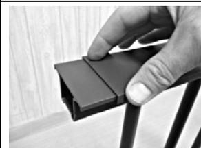
10. At the point(s) where you installed support block connectors (step 2), carefully measure the distance from the underside of the bottom rail (B) to the floor. Cut support block material (F) to fit. Remove rail assembly from the saddle brackets (C). Slip support blocks over support block connectors (G). Slide the rail back into place and make certain the rail is plumb.
