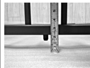
11. Slide and hold the bottom bracket (D) firmly against the post or wall. Secure the bracket with self-drilling screws (H). Repeat the process on the other side.
