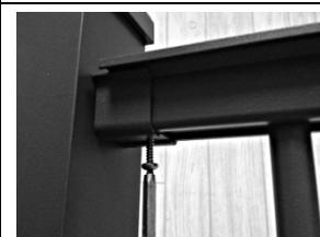
13. If a deck board is to be installed on top of the rail, carefully measure and cut the material to the length required. Place the deck board on top of the rail and secure from the under-side of the rail as shown, with the appropriate fasteners under the flange of both sides of the rail.
