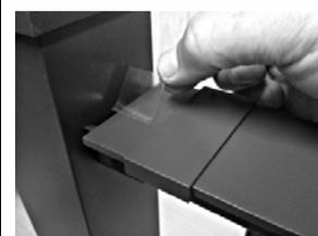
*Note: This photo depicts a fully assembled rail section installed between two posts, with a deck board mounted on the top rail. The left side is butted up to the post and the right side is depicting an application where the post may be cut flush with the top rail for a continuous board to be mounted over the post and provide an uninterrupted sight line.*
