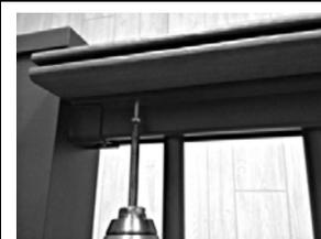
14. If the deck board will not be installed, place the adhesive tab (J) to the top surface of the top rail (A) near the post. Slide the top rail cap (E) towards the post and press down to secure it with the adhesive tab (J).
