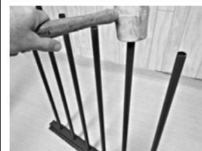
4. Attach balusters to bottom rail (B) beginning at one end and working to opposite end. Stand the assembly upside down on the surface of the box and firmly tap the bottom rail with a rubber mallet to secure the balusters in place. Stand assembly upright.
