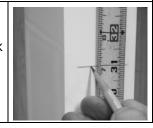
6. Align screw holes in the upper and lower saddle brackets (C&D) on the marked lines. Make sure the brackets are centered on the posts. Mark the screw hole locations with a pencil.
