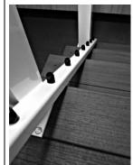
2. When the final position is determined for the post, mark the hole locations of the four 3/8" diameter mounting holes provided on the base and remove the post assembly. Drill the marked locations into the decking and reinforcement using the proper size drill required for the fasteners being used.
